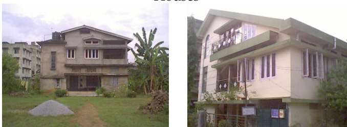
Figures 1.4 Conventional Housing - Multilevel RC framed houses with light roofing
