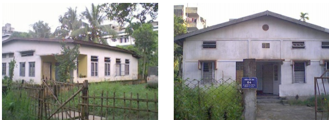
Figures 1.2 Conventional Housing - Confined Masonry Houses
